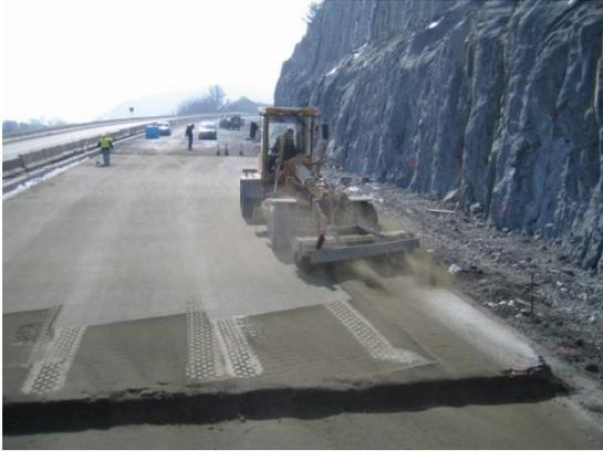
*Figure 4: making of the exposed aggregate surface*
